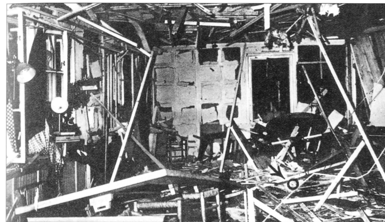
Above: The wreckage in the conference hut in Rastenburg after Stauffenberg's bomb had exploded. Hitler's life was primarily saved by the flimsy construction of the building whose open windows dissipated much of the blast. As a result he sustained only superficial injuries.
